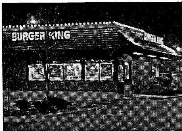
▲ Outlining the perimeter of commercial buildings.
